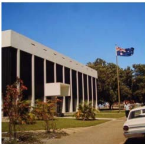
Figure 13 – The Reserve Bank of Australia building, Darwin, c1970. Source: National Archives of Australia.
