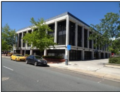
Figure 20: South West View
