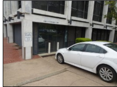
Figure 24: Former Delivery Dock Location
