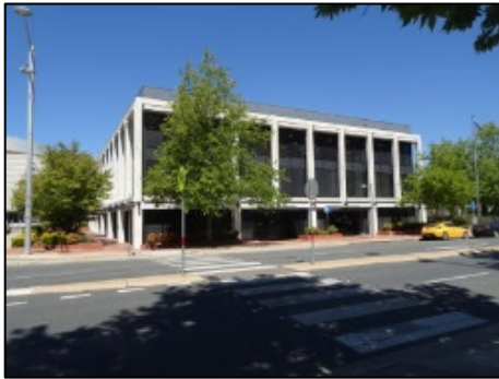
Figure 16: View of RBA Building and Precinct from North West
