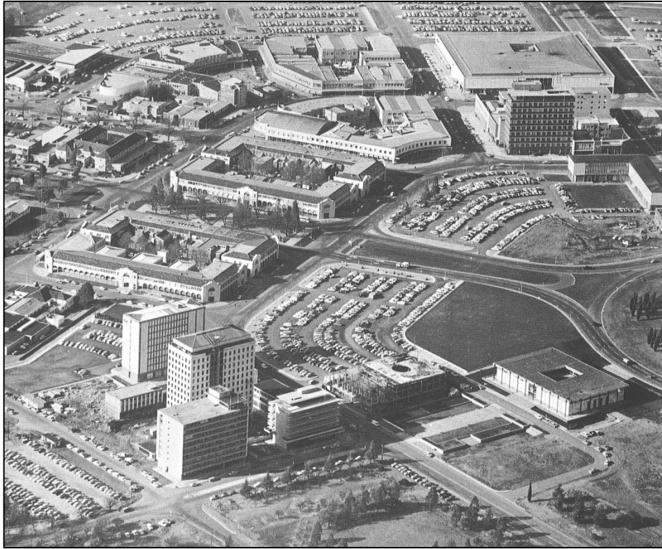
Figure 5: Civic Circa 1964 Showing RBA Building Under Construction
