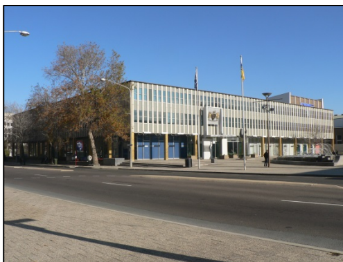
Figure 46: Civic Square Buildings
