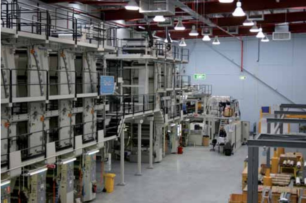
Securrency's new polymer substrate line, commissioned early in 2007, has doubled its production capacity.
