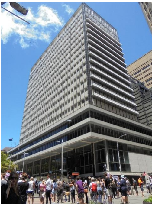
Figure 12 – General view of the northwest corner of the Head Office building.
