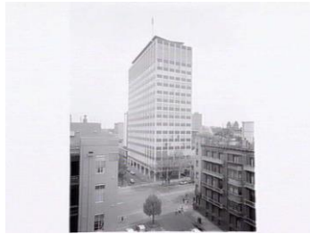
Figure 39 - The Reserve Bank of Australia, Melbourne, c1967.
