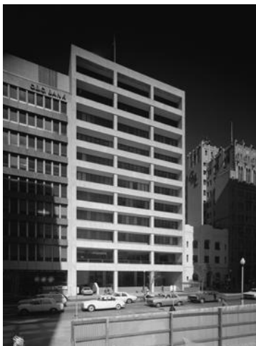
Figure 41 - RBA building, Perth, formerly located at 45 St George's Terrace. Source: State Library of Western Australia http://www.slwa.wa.gov.au/images/pd224/224034PD.jpg , Fritz Kos
