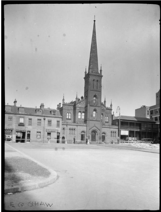
Figure 54 - Phillip Street buildings demolished to form the eastern extension of Martin Place, photographed by EG Shaw, 1935. St Stephen's Church and the building to its right, St James Parsonage, were subsequently acquired by the Commonwealth of Australia for the RBA Head Office building.
