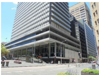
Figure 33 - View of the northwest section of the RBA building from the corner of Phillip Street and Martin Place.
