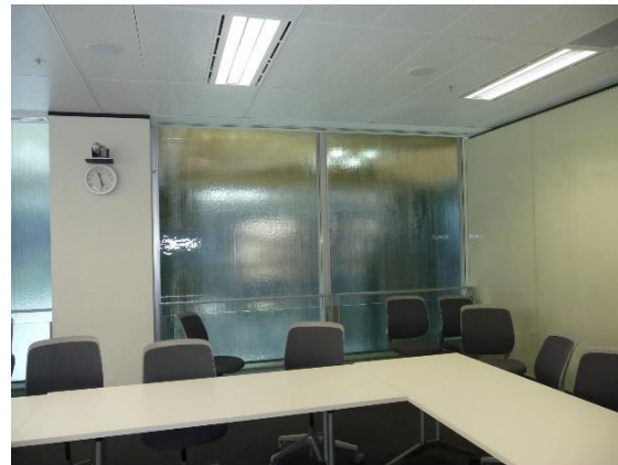
Figure 22 - Typical Mezzanine office fit out. Note the full-height textured glass forming the north wall of the mezzanine level is visible from within the ground floor vestibule.
