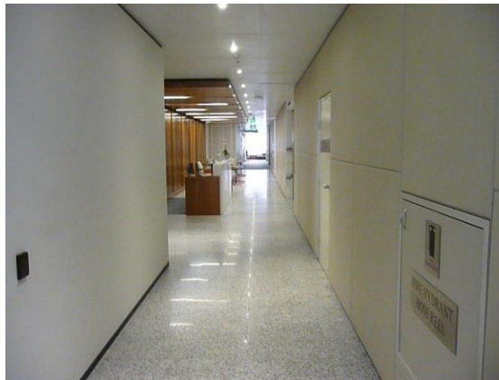
Figure 21 – Typical finishes installed in 2014 in the corridor and reception area located at the Mezzanine Level.
