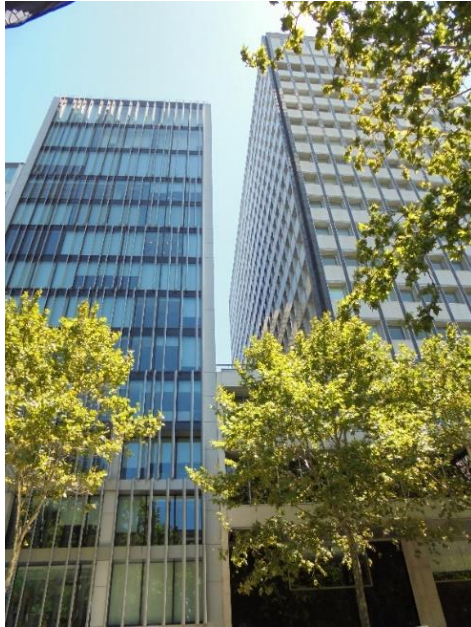
Figure 14 - Oblique view of the south elevation of the RBA Head office building.
