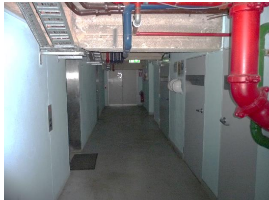
Figure 27 - Main east-west corridor located at Level 18 looking west.
