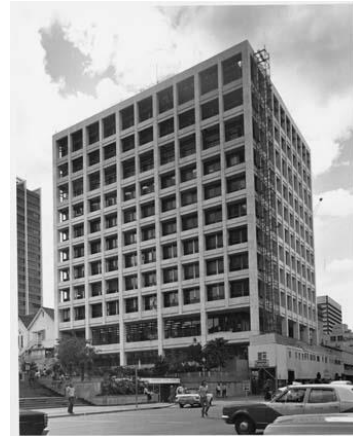
Figure 37 - RBA building, Brisbane. Source: NAA
