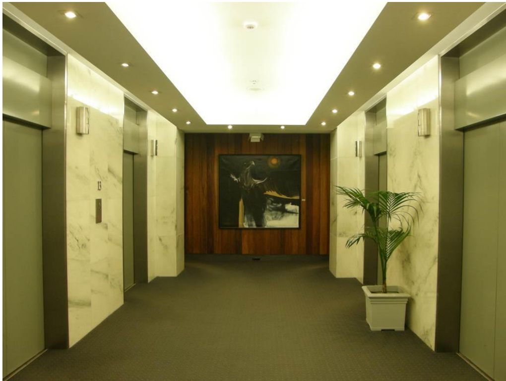
Figure 47 - Typical office level lift lobby showing original (1964) marble wall finishes and timber wall panelling. The original ceiling was replaced c2000.
