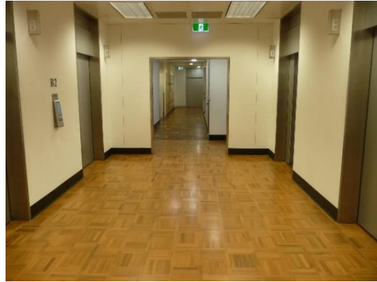
Figure 19 – Typical painted rendered finishes at Basement Levels 1 and 2.
