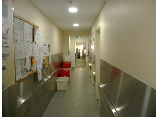
Figure 25 - Level 16 service corridor, looking east to kitchen.
