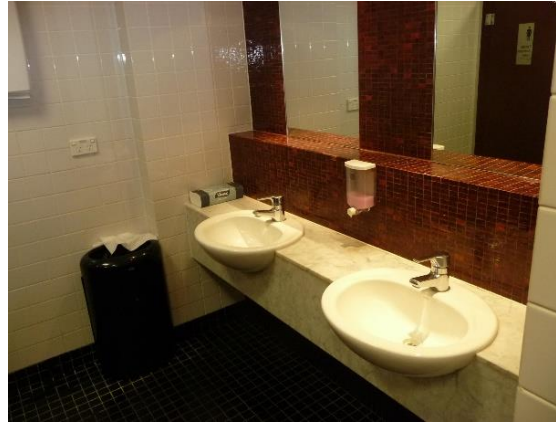
Figure 17 – Photograph of typical refurbished lavatory areas throughout the RBA building.
