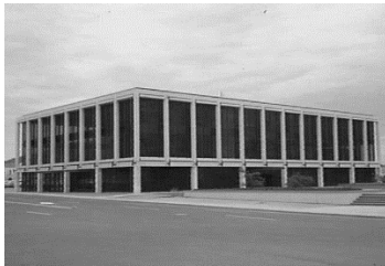
Figure 38 - The Reserve Bank of Australia, Canberra, c1964.
