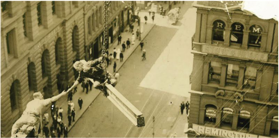
From the Reserve Bank's archival photographic collection, an image of the construction of the Commonwealth Bank of Australia's head office premises titled 'Lend us your hammer Jim', December 1914; RBA Archives PN-000685
