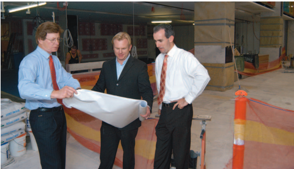
Paul Barry, Information Department, and Ed Jacka, Facilities Management Department, review progress on the construction work for the Museum, with one of the outside contractors (centre).
