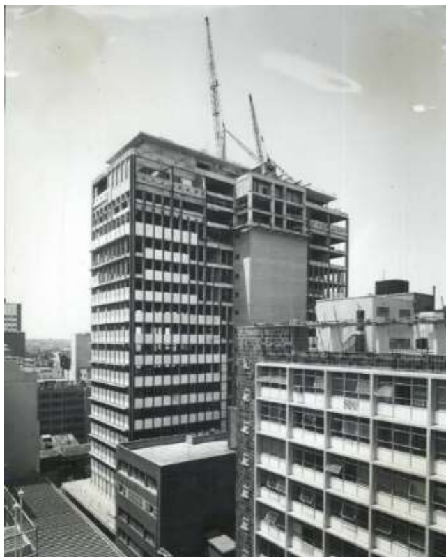
Figure 3 – View of the steel framed construction of the Reserve Bank of Australia Head office building, c1962. Source: National Archives of Australia
