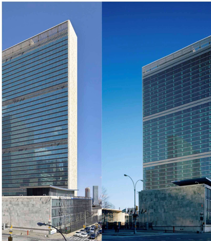
Figure 32: UN Secretariat Building, New York. The west elevation before (left) and after (right) renovation. The original transparency and hue were restored (Source: DOCOMOMO US and Heintges & Associates, United Nations Headquarters Campus Renovation of Facades, 17 April 2017, https://docomomo-us.org/news/united-nations-headquarters-campus-renovation-of-facades )
