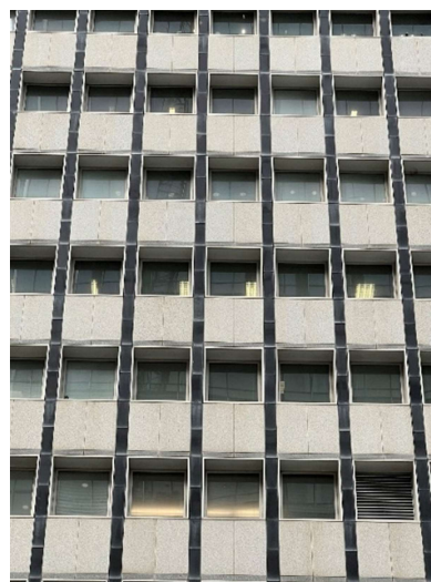
Figure 24 - View of the later overclad replicating the original layout pattern below. The relationship between the narrow, dark verticals and alternating horizontal bands of windows and lighter stone panels that create the 'tartan' effect is clear. (Source: NBRS 2023)
