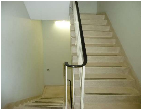
Figure 24 – Example of fire stair finishes and painted steel balustrades within the RBA Head office building.
