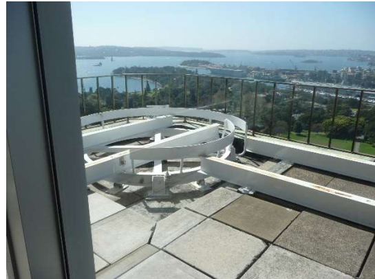
Figure 37 - General view showing the concrete pavers and access equipment for servicing the exterior of the RBA building.
