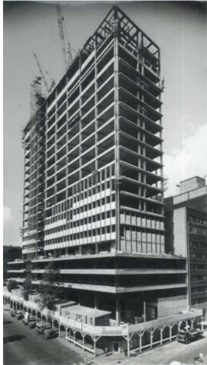
Figure 5 -View of the northwest corner of the RBA Head Office showing the original marble panels being installed to the north and west elevations, c1962. Source: National Archives of Australia.
