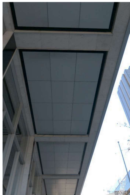
Figure 21 – General view of the podium soffit adjacent to the north side of the RBA Head Office entry. Note the original suspended marble soffit was replaced in c2001.
