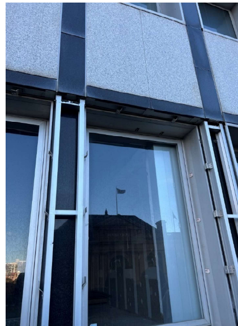
Detail of where the overcladding to the head and reveal of the windows has been removed. Then secondary frame used to support the overcladding pushes out the face of the building, and the depth of the reveal, in the order of 100mm.
