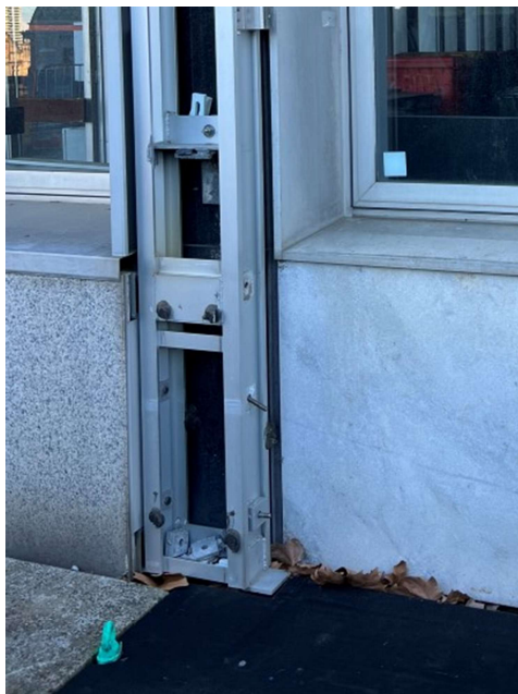
Detail on the western façade where a portion of the 1990's overcladding has been removed revealing the original sill profile and stone panel (to the right of the overcladding support framing)
