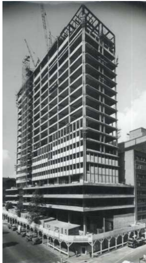
Figure 6 -View of the northwest corner of the RBA Head Office showing the original marble panels being installed to the north and west elevations, c1962. Source: National Archives of Australia.
